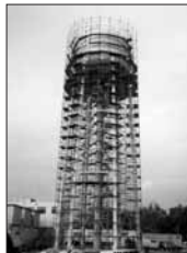
Atlantic erects challenging scaffolding around structures such as this water tower.
