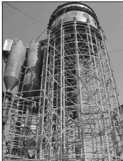
When a Gulf Coast refinery was hit by Hurricane Rita, Atlantic's scaffolding withstood the 150-mile-per-hour winds.
